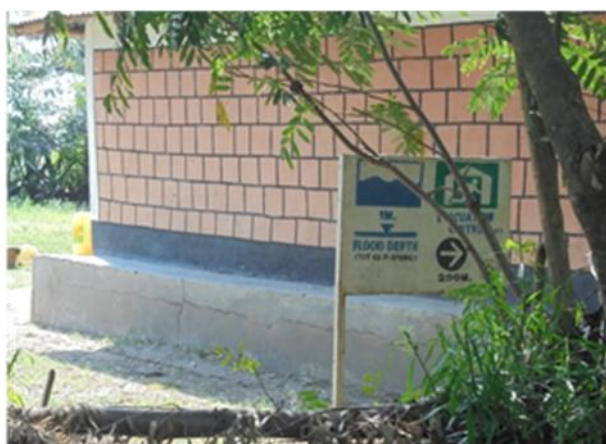
Figure 13. Raising of floor above flood level in Nyamasaria.
