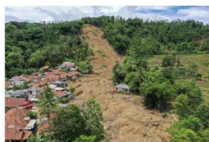
Figure 1. Open field prone to landslides
