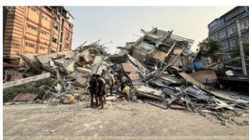
Figure 2. Impact of the Myanmar Earthquake
