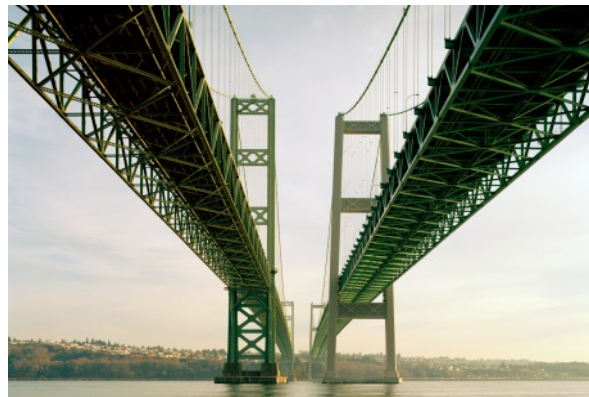
Figure 15. The new Tacoma Narrows Bridges.
