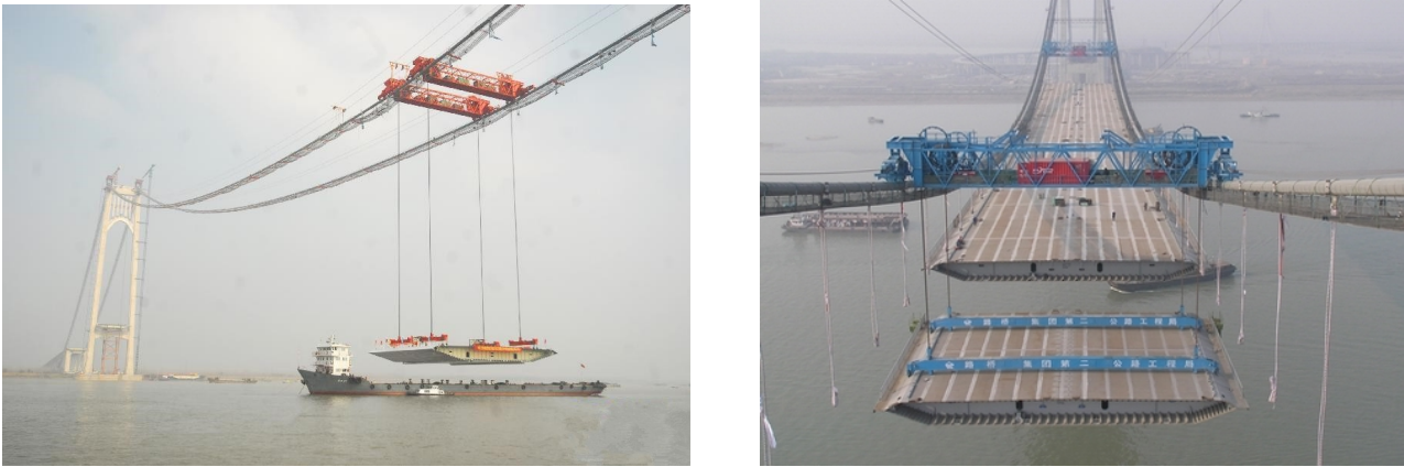
Figure 16. Rectangular deck segments for the erection of a suspension bridge.
