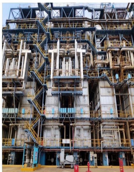
Figure 1. External structure of ethylene cracking furnace.
