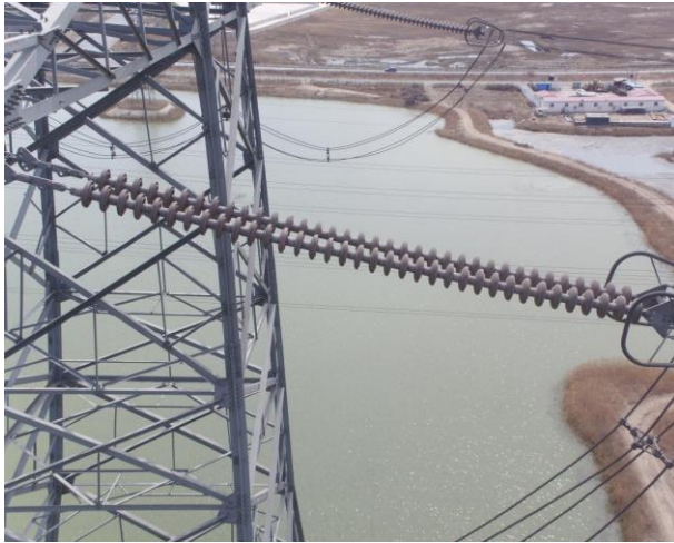
Figure 25. Raw image of a tower structure.
