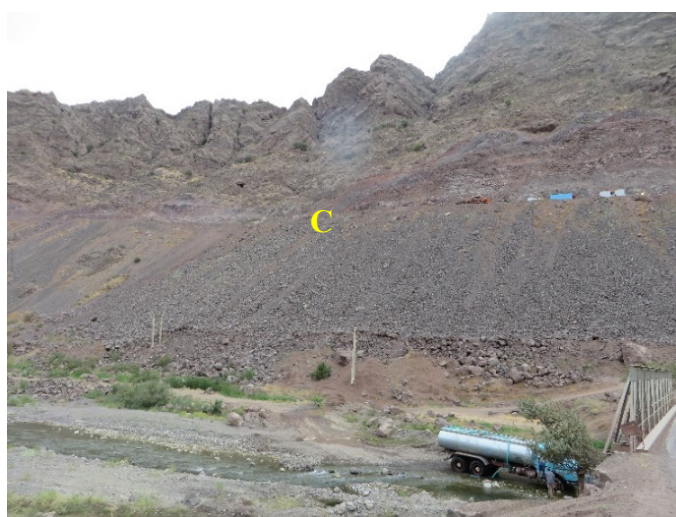
Figure 3. Anthropogenic colluvium (C) produced by surface mining (north flank of Shahrud River, northern Iran). Waste dumping may increase slope instabilities or cause other geoenvironmental problems.
