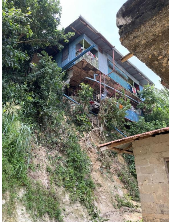
Figure 11. Picture of a poorly constructed house built on a slope, taken by participants from Mkoani during the photo elicitation activity.
