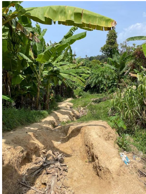
Figure 12. Picture of a damaged, unpaved road connecting local villages to the main road, taken by participants from Mkoani during the photo elicitation activity.
