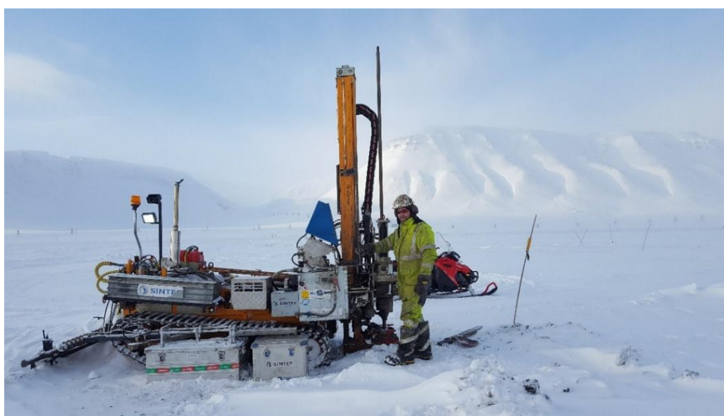
Figure 2. Geotech 504 drilling rig of SINTEF during operation in Adventdalen .
