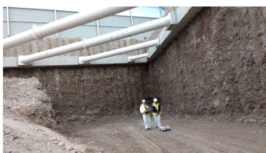
(a) GPR acquisition along a longitudinal profile.
