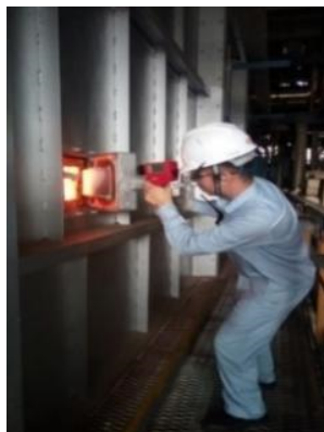
Figure 1. Measurement of the outer-surface temperature using a thermoprobe.
