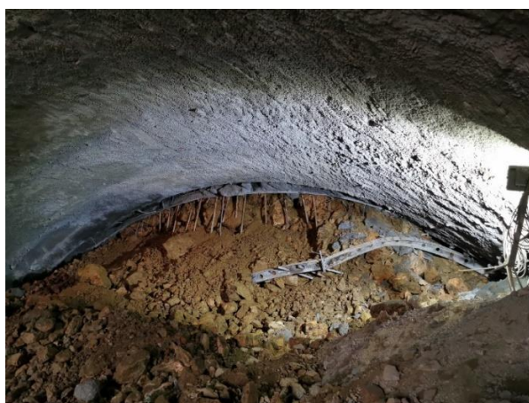
Figure 9. Tunnel collapse.
