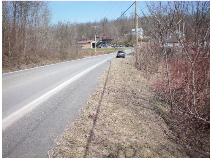
Figure 5. Photograph showing the topography of the Barnerville Road (A-A') traverse.
