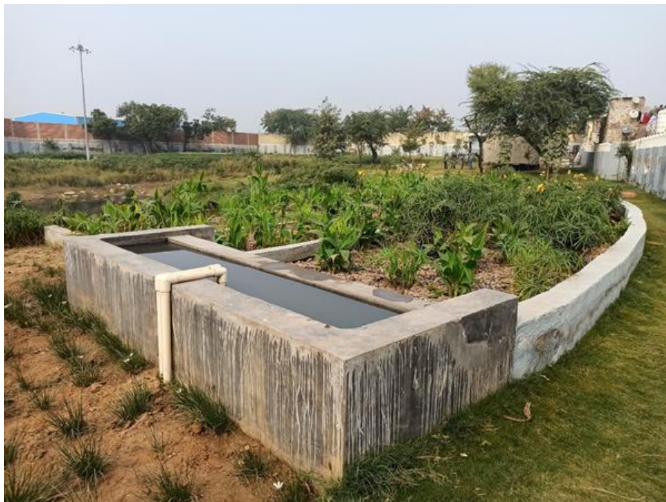
Figure 3. Gravel bed with wetland plants to treat biodigester effluent.
