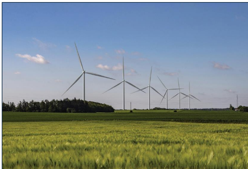
Figure 1. The wind farm under study.
